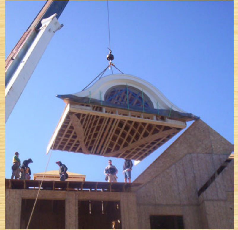
Ready to Install
