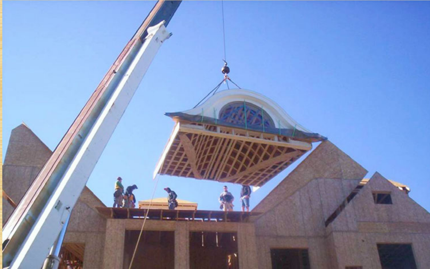
Photos: Reliable Truss and Components | Jobsite Installation
