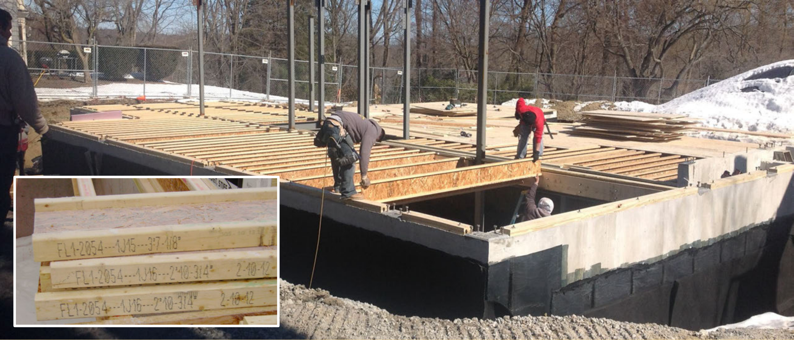
Photos: National Lumber | Precision End Trimmed I-Joists Being Installed by Builder's Crew – Available with Inkjet Printing for Planned Installation
